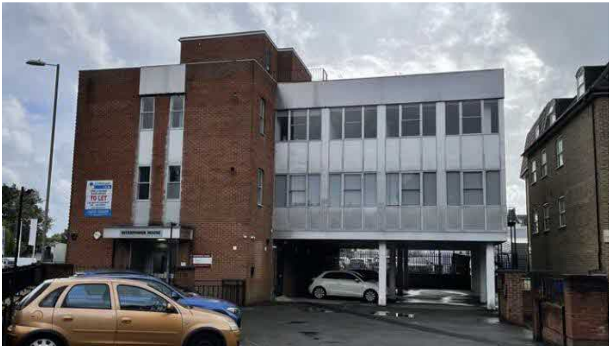
Figure 2 View towards Interpower House from the north, looking south
