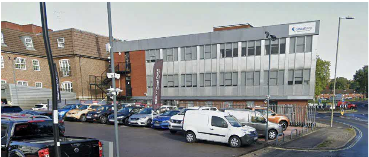
Figure 4 View of Interpower House from the south
